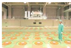
JNFL Vitrified Waste Storage Center and HLW storage pits (photos: courtesy of JNFL).
