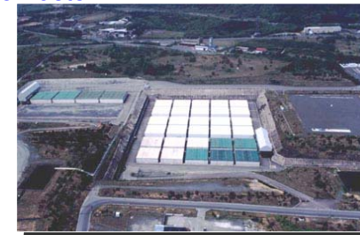
(Low Level Radioactive Waste Disposal Center at Rokkasho)
